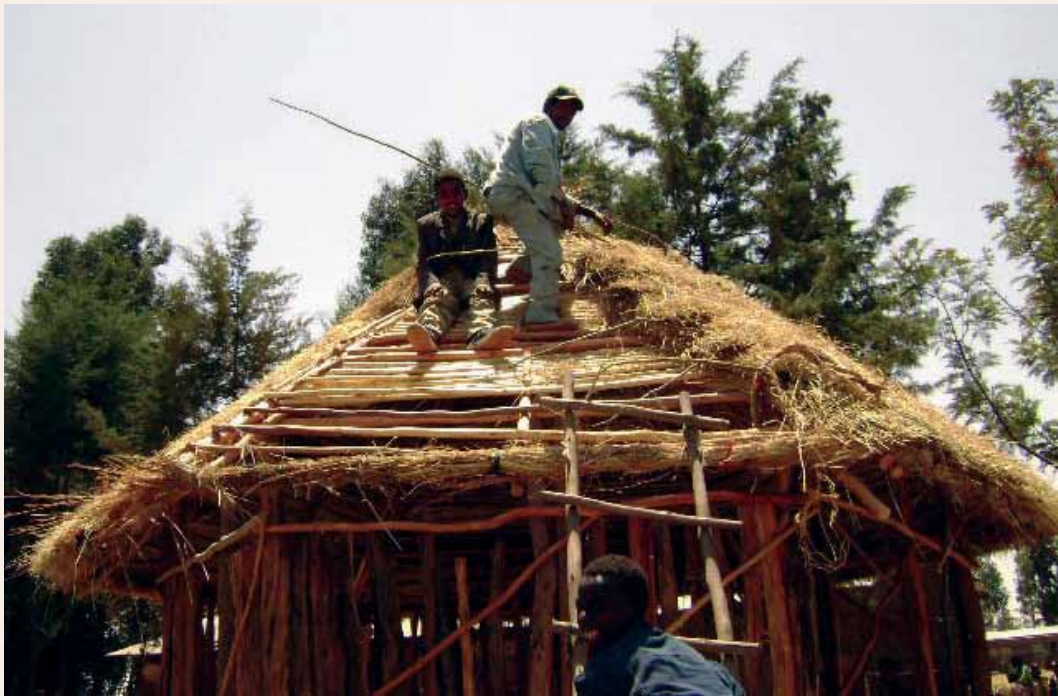
Construction of a learning centre at a school
